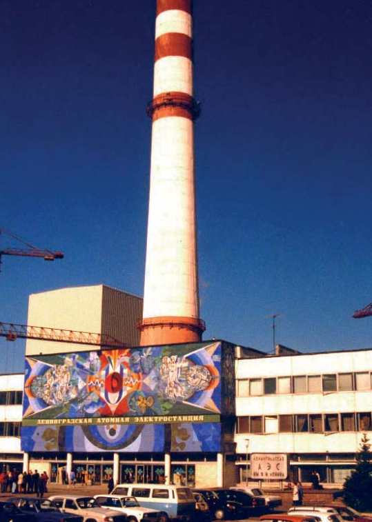
The Nuclear Power plant "Leningrad" near St. Petersburg. Photo: Norwegian Radiation Protection Authority
