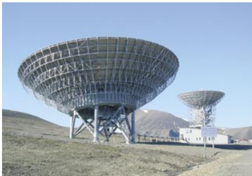
EISCAT Svalbard Radar. Photo: EISCAT Association
