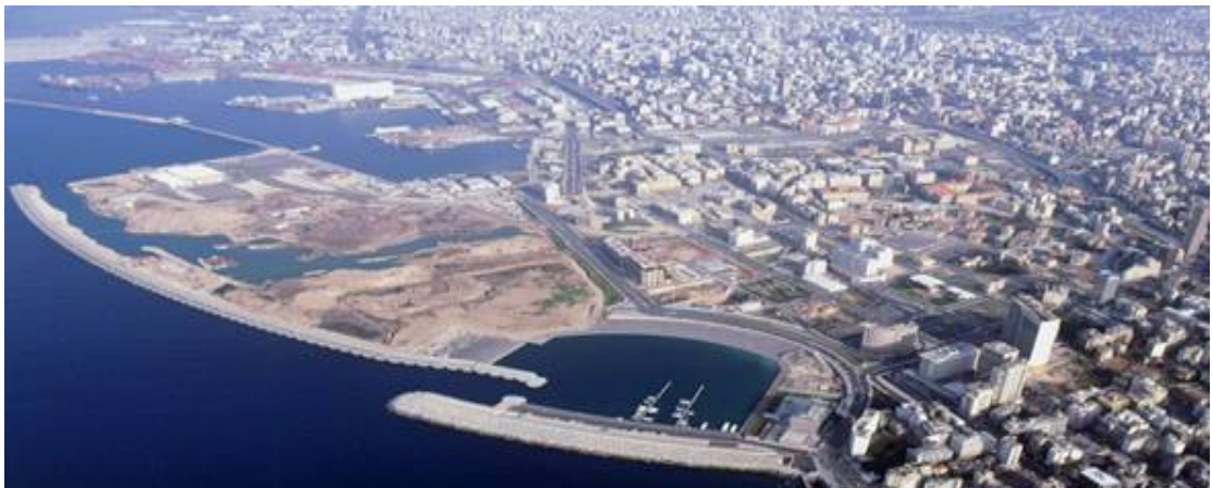
FROM: THE URBAN HUB: Aerial view of Postwar Beirut's landfill and urban void of the central district Looking North East with a full context of Quarantine top left, 2004. The current waterfront landfill of Quarantine, being occupied by the Port Authorities and facilitates in part as Military Base.
