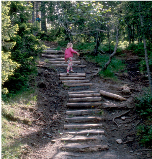
Building walking paths to prevent erosion will become more important as climate change will lead to heavier precipitation in large regions of Norway. Here from Estenstadmarka, Trondheim. Photo: Mari Lise Sjong
