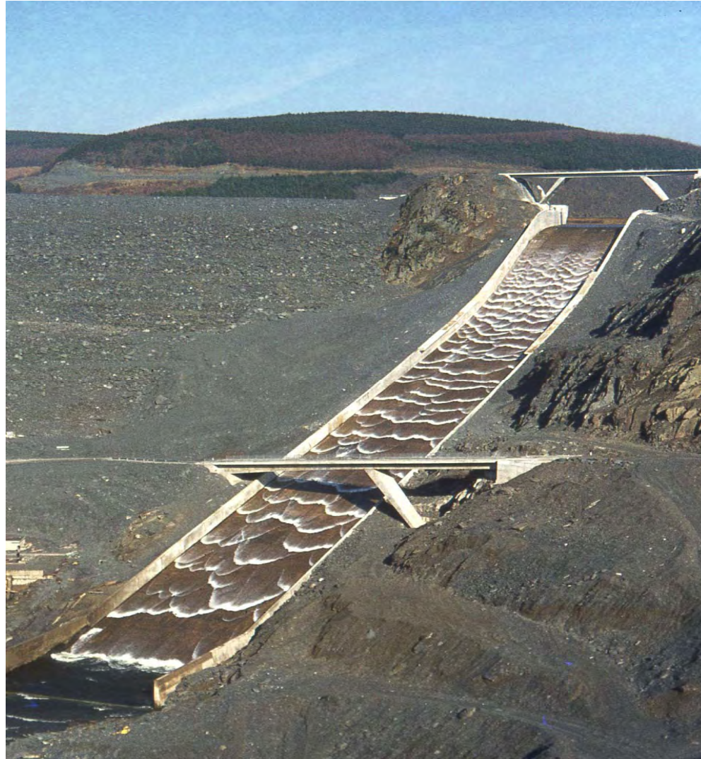
Spillway from Llyn Brianne Dam, Wales
